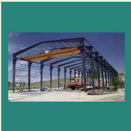
Pre Engineered Building Structure
